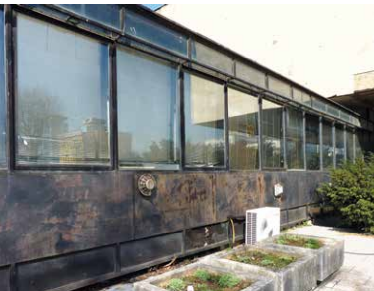
Steel construction with obvious and very advanced corrosion; stone surfaces also showing severe damage (photos 2016)
